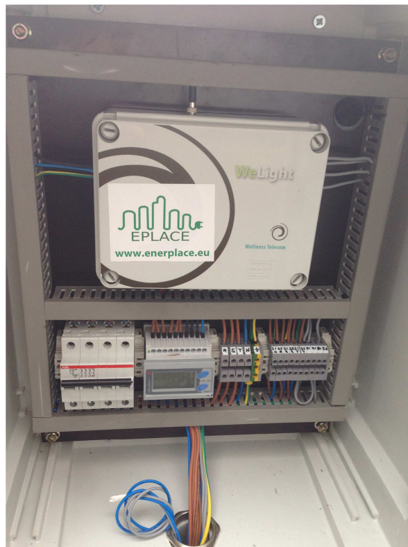
Figure 2: Welight installation in Cartaya
